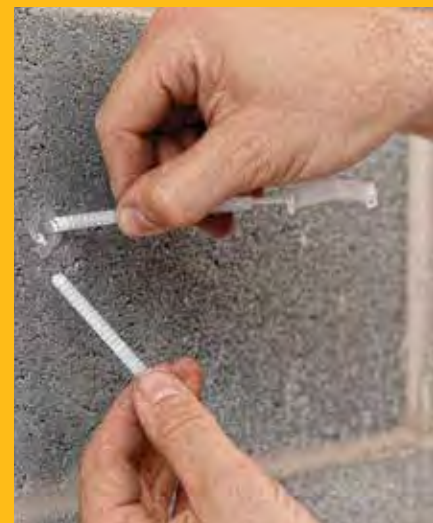
STRAP-TOGGLE INSTALLATION
